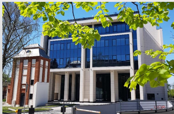
ALCHEMIUM – new building of Faculty of Chemistry of Lodz University of Technology (photo by J. Szabela)
